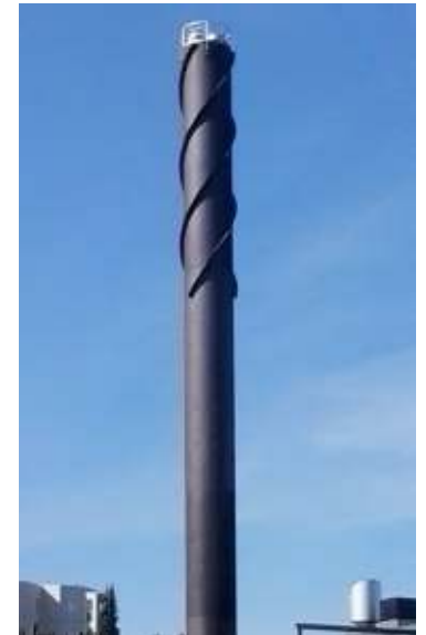
The reason for spiral vortex breakers on industrial stacks
