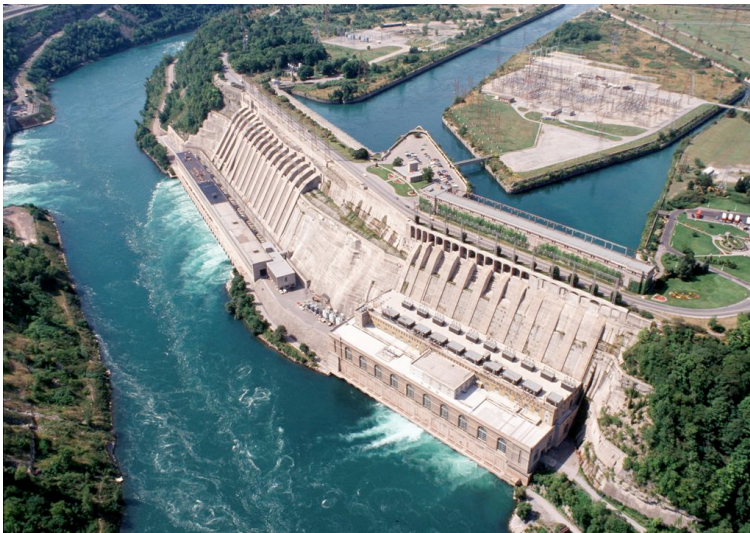
Sir Adam Beck Hydroelectric Power Station (Niagara Falls)
